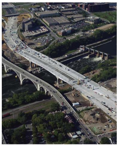
was removed, the less scour, but designers did not want to remove more than was necessary. The scour analysis allowed the designers to determine how much of the old pier needed to be removed without causing too much scour on the new bridge pier.
